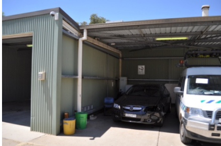
Figure 6 Existing van dock to be demolished
