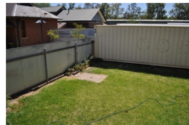
Figure 9 Existing service pit to be capped and removed
