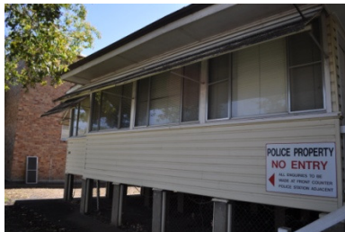
Figure 4 Existing weatherboard offices to be retained
