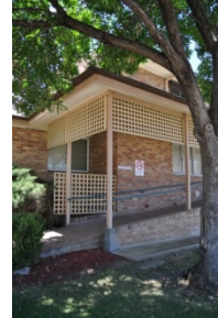
Figure 7 Existing entry ramp to be amended
