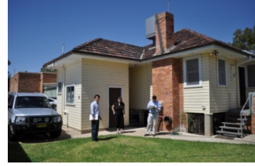
Figure 11 Existing weatherboard building to be demolished
