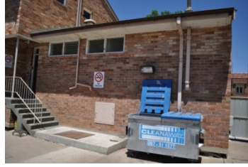
Figure 10 Existing portion of brick building to be demolished
