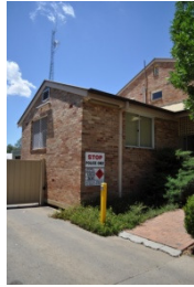
Figure 2 Existing single storey brick building to be demolished
