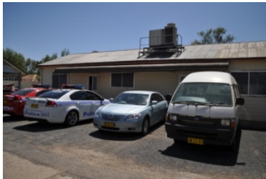
Figure 12 Existing weatherboard building to be demolished
