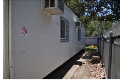
Figure 3 Existing demountable to be retained
